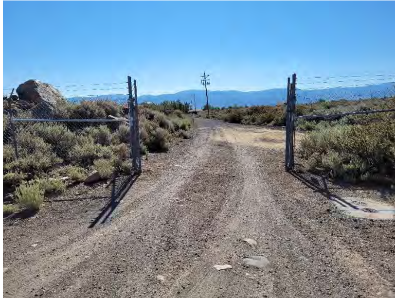
Figure 5. Existing Perimeter Chain Link Fence
