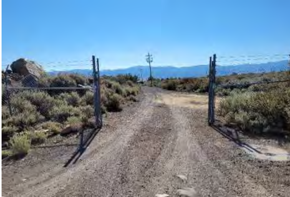
Existing Perimeter Chain Link Fence
